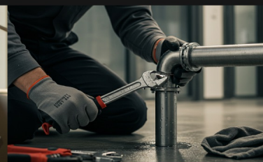
On-site team responds to the incident
